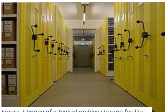
Figure 2 Image of a typical archive storage facility. National and local record offices are required to have facilities which align with the British Standard 5454.
